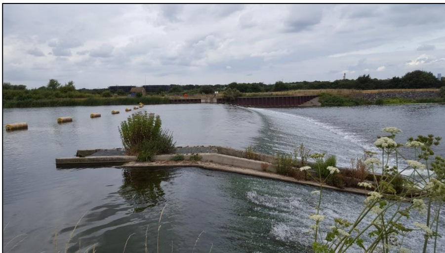
Plate 4-2 - An example of a typical water level control structure.
