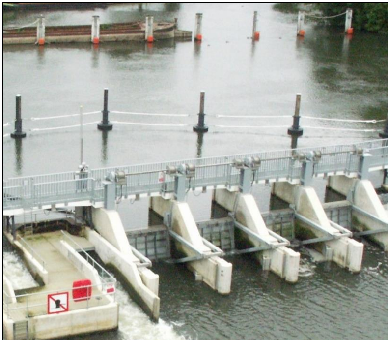
Plate 4-1 - An example of a typical flow control structure.
