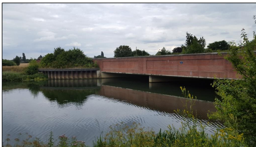
Plate 4-3 - An example of a typical culvert.
