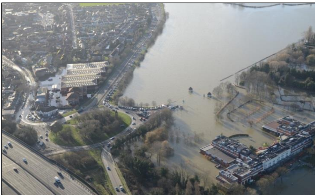
Plate 1: Flooding at Runnymede (M25 junction 13) in 2014
