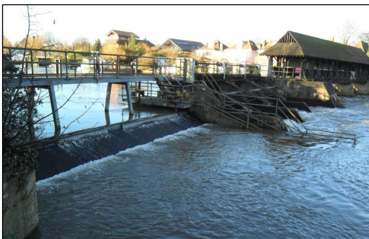
Plate 4-5 - Photograph of the existing overfall weir (far left) on weir C at Molesey.
